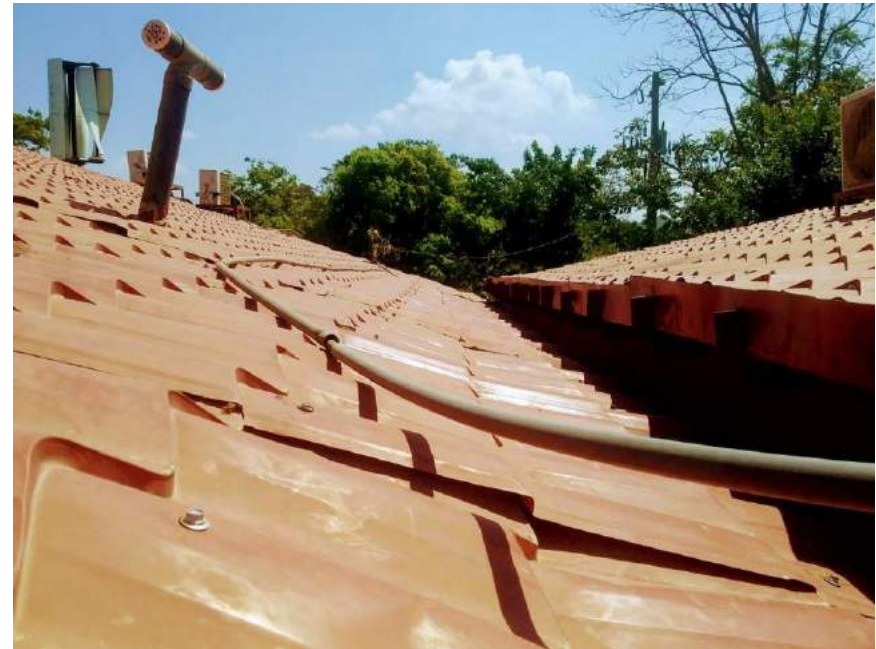
Roof damage recovery
